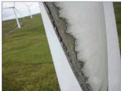
Figure 1: Typical blade damage because of Leading Edge Erosion
