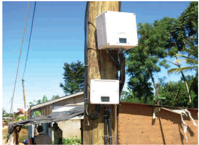
JUMEME power meters for a mini-grid in Bwisya village, Ukara island, Tanzania
