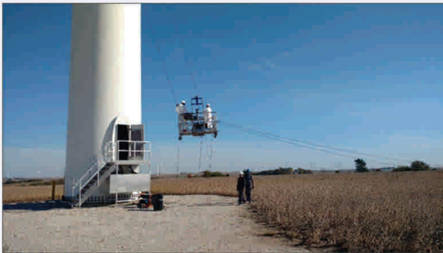
Figure 5: Platform on its way to the damaged blades
